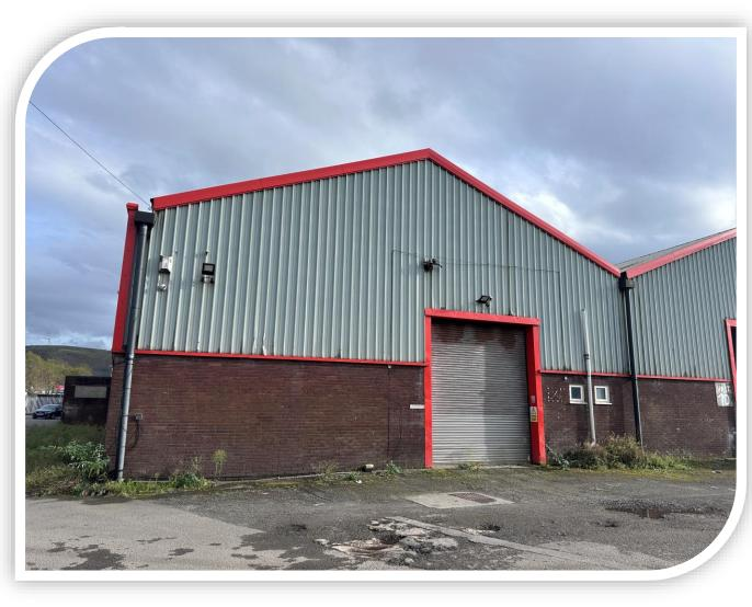
Minimum eaves – 5.79m Roller shutter – height – 4.20m Width – 3.618m
